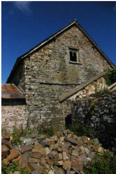
Building 1: The probable late medieval detached kitchen block.
