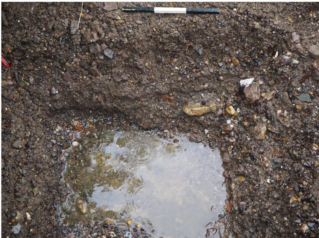
*Figure 4 – This photo was taken approximately 30 seconds after the one above (Fig 3) and illustrates the rate that water was ingressing into the trench.*
