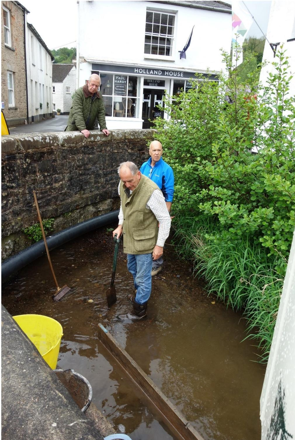
The flow of the leat was reduced and Phillip Hull constructed a small cofferdam around the area to be excavated. Whilst the amount of water entering the area of Trench 3 was greatly reduced, it proved impossible to prevent the ingress of water into the trench.
