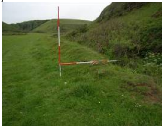
Figure 23: Earth bank against the west edge of 'Swan Pool' enclosure
