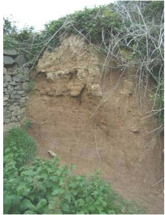
Figure 15: H2 showing the compacted earth infill layers (east)
