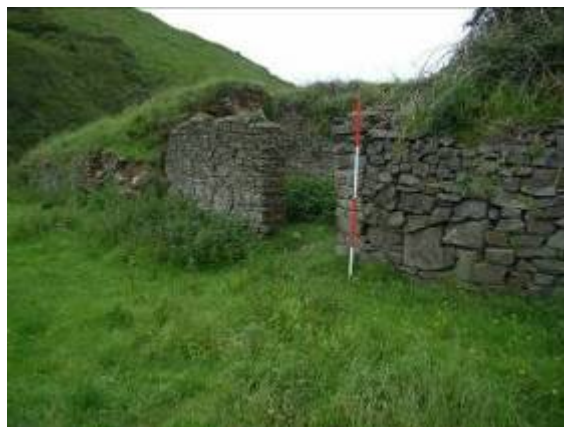
Figure 13: H2 Inserted cattle shelter on south east face
