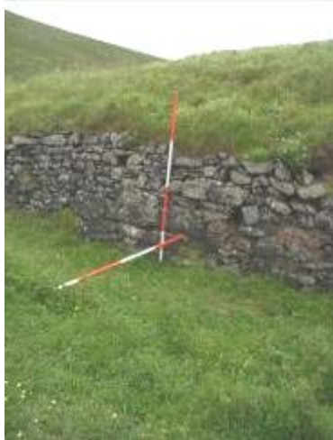
Figure 8: H2 viewed from north west
