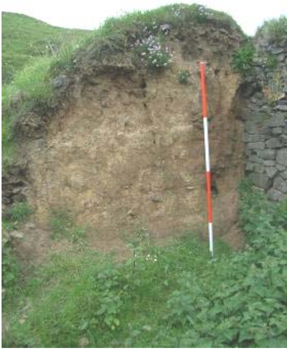
Figure 14: H2 showing the compacted earth infill layers (west)
